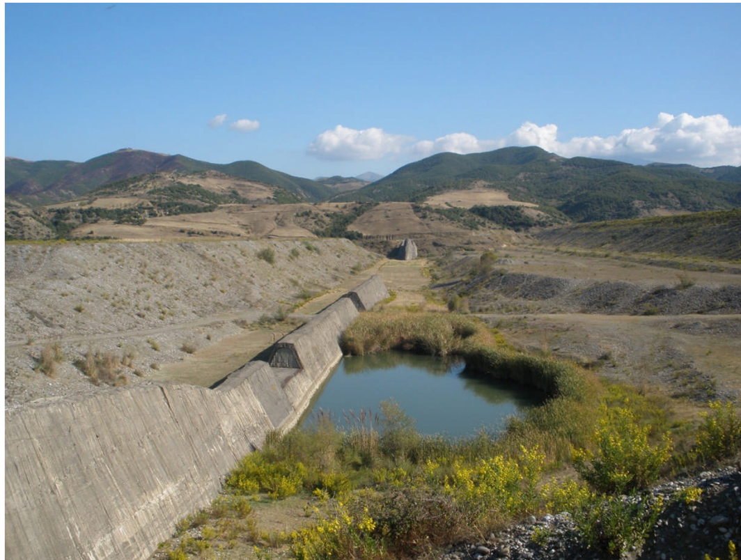
Dam, View from the left abutment
