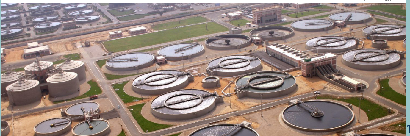
Gabal el-Asfar treatment plant in Egypt.
