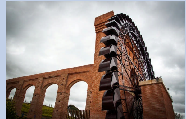
Mountain weir (Aranjuez, Spain)
